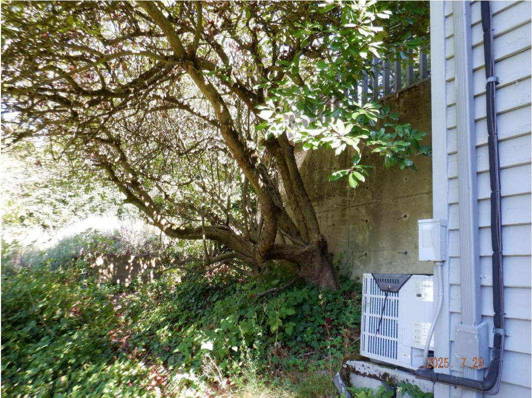
Mature photinia shrubs adjacent to concrete wall below deck
